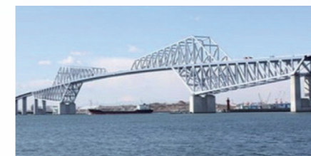
Tokyo Gate Bridge
