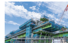
Yodogawa Higashi Viaduct on the Keihan Electric Railway
