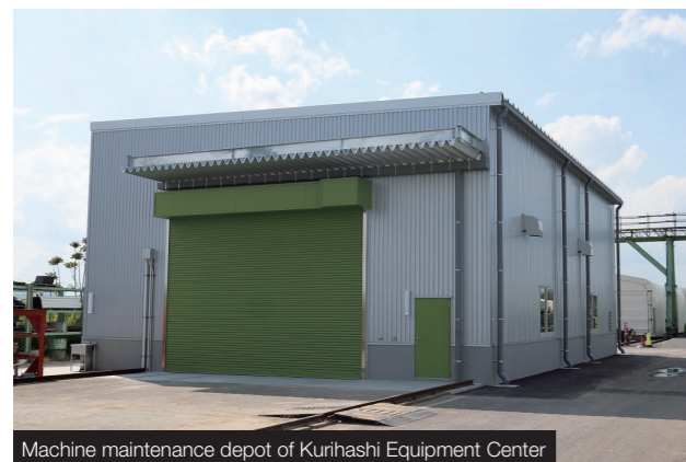
Machine maintenance depot of Kurihashi Equipment Center
