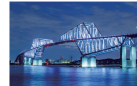
Tokyo Gate Bridge
