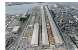
Chiba Works of MIYAJI ENGINEERING CO., LTD.
