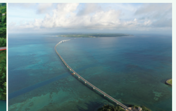
Irabu Ohashi Bridge/Miyakojima City, Okinawa Prefecture
