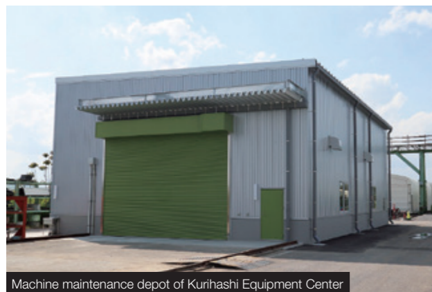
Machine maintenance depot of Kurihashi Equipment Center
