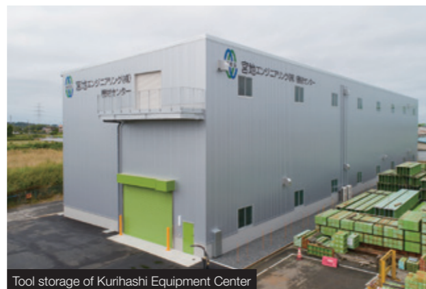
Tool storage of Kurihashi Equipment Center
