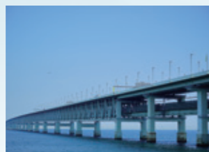
Kansai International Airport Access Bridge (Sky Gate Bridge R)
